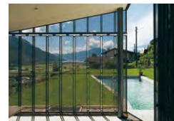
Private Residence, Tessin, CH Davide Macullo, Lugano, CH Torsetta SA Lattonieri, Muralto, CH TECU® Classic_flatmesh
