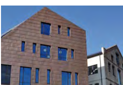
Granary Wharf - Abbey Road, Barking, UK Pollard Thomas Edwards Architects (PTE), London, UK Roles Broderick Roofing Ltd, Chobham, UK TECU® Bronze
