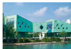
Yefei's Creative Street, Shanghai, SG Will Alsop Architects, London, GB; U/Jiang Architects & Engineers, Shanghai Hanchang Industrial Development Co., Shanghai TECU® Patina, TECU® Oxid, TECU® Bronze
