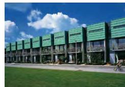
Residential building, Purmerend, NL Roy Gelders Architecten, Amsterdam Ridder Dak- en Wandsystemen BV, Hoorn TECU® Patina
