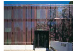
Office building of the International Ice Hockey Federation, Zurich, CH Tilla Theus und Partner AG, Zurich Scherrer Söhne AG, Zurich TECU® Classic_flatmesh
