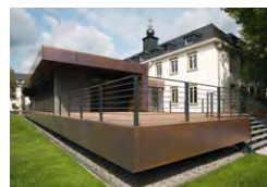
BMAS, Canteen Building V, Bonn pbr, Planungsbüro Rohling AG, Osnabrueck KME Architectural Solutions, Osnabrueck TECU® Classic_bond
